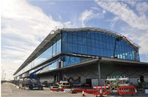
At 350m long and 45m wide, concourse C consists of twelve aircraft stands with the option of a further two stands safeguarded for the future. With a semi-unitised façade provided by MERO-SCHMIDLIN (UK) PLC towering 16m above the apron level, the design matches the other two buildings manufactured by sister company Schmidlin of Switzerland.
